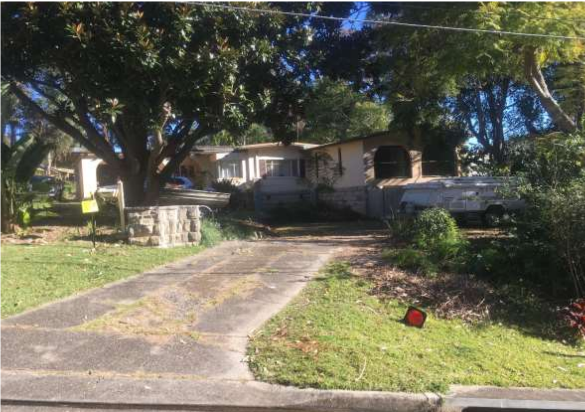
Figure 4 : 163 Darley Street West (double block)
