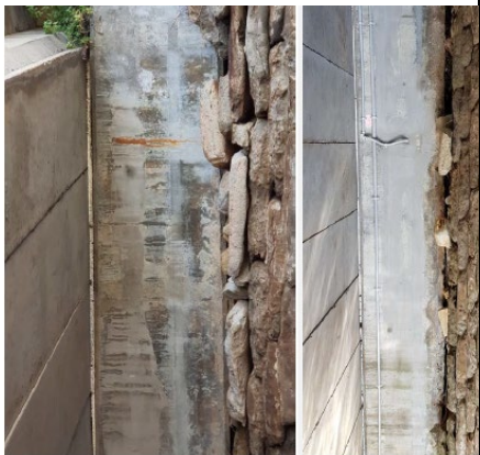
Photo No: 26 Abutment 2 Photo No: 27 Ab Evidence of corrosion staining under unit 28. Evidence of possible settlement
