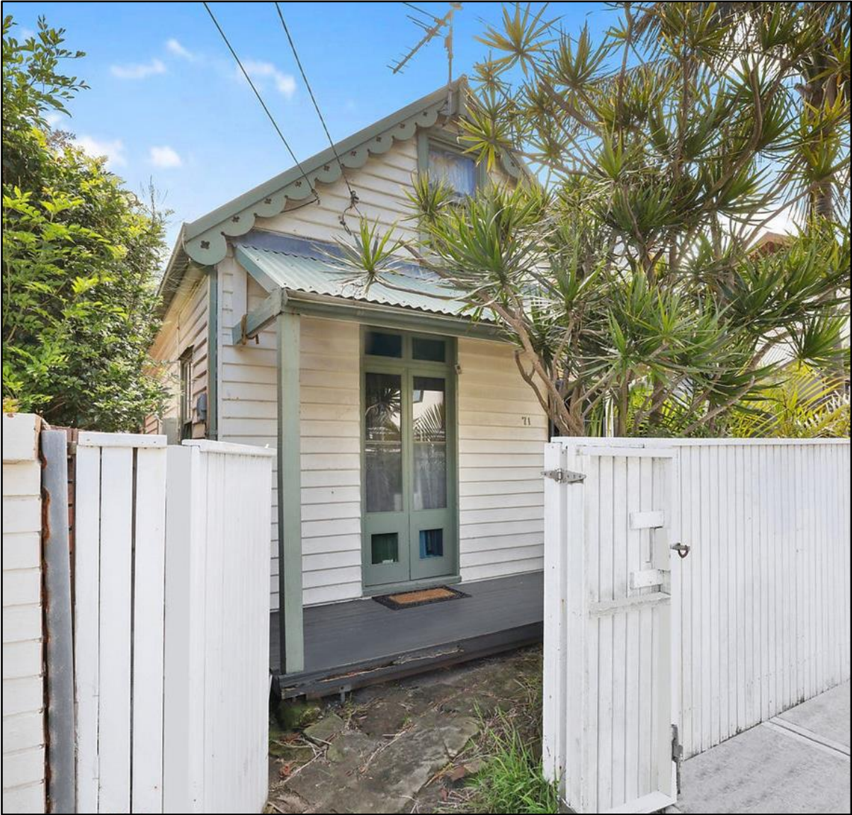
Figure 2: View to the front facade of the subject site
