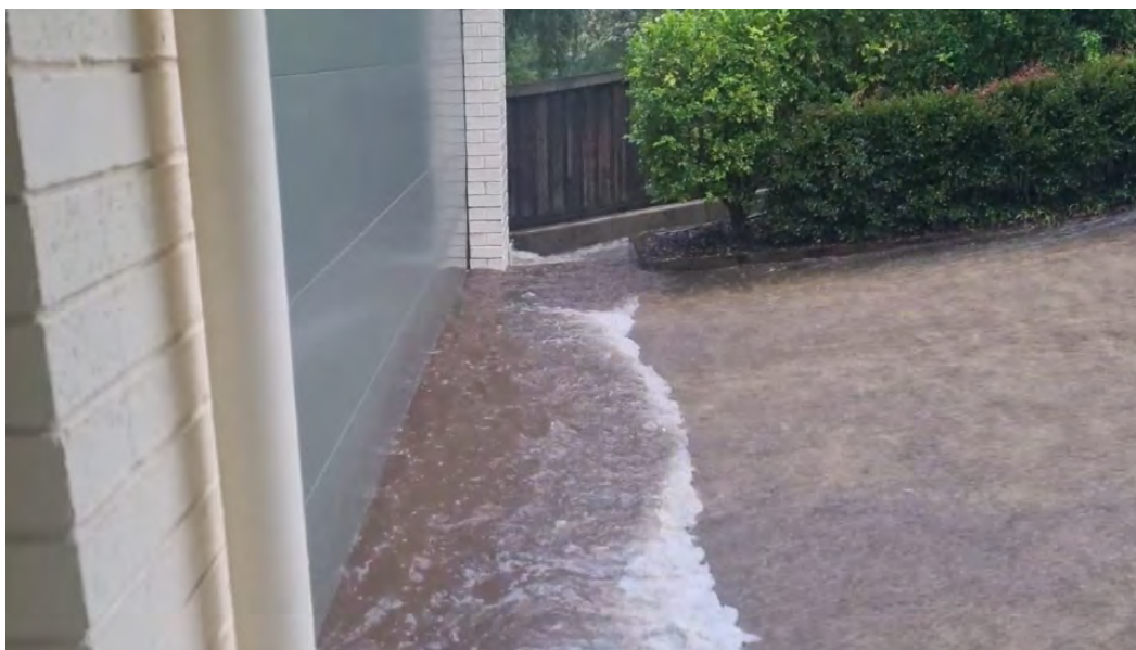
Photo 35: Example of water ponding against a building (MH_576)
