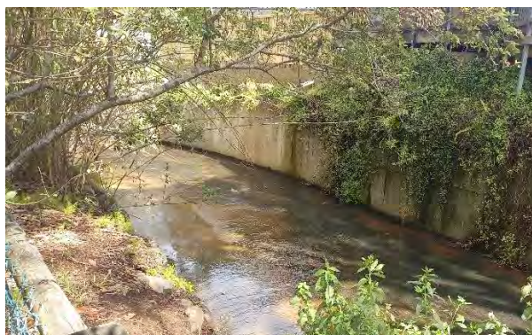
Photo 5: Frenchs Creek concrete channel section parallel to Calool Crescent
