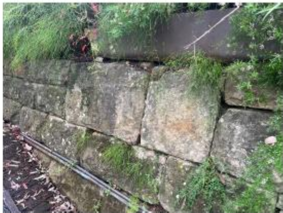
Figure 155: Close view of stonework showing drystone construction
