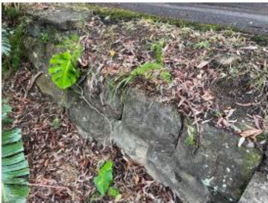
Figure 154: Two courses of stonework below Clavering Road
