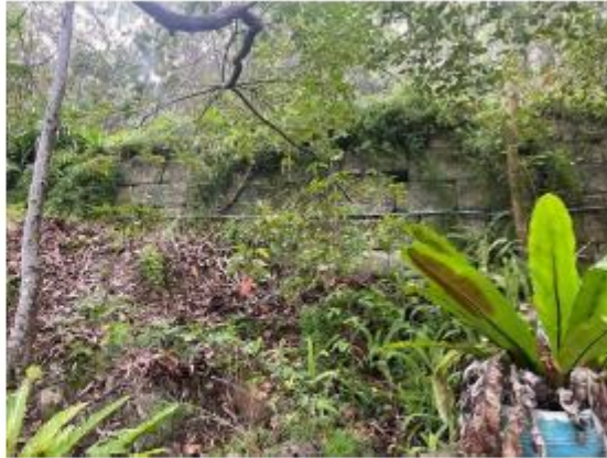
Figure 153: Stone wall supporting Clavering Road, showing dense surrounding vegetation
